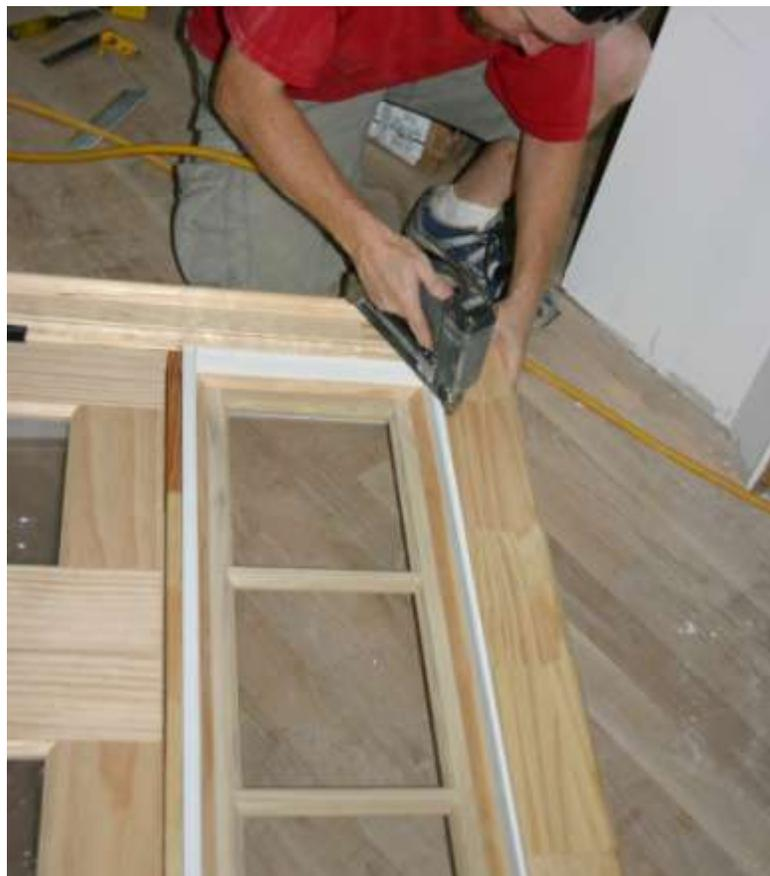
Complete casing installation on one side of transom / door unit
