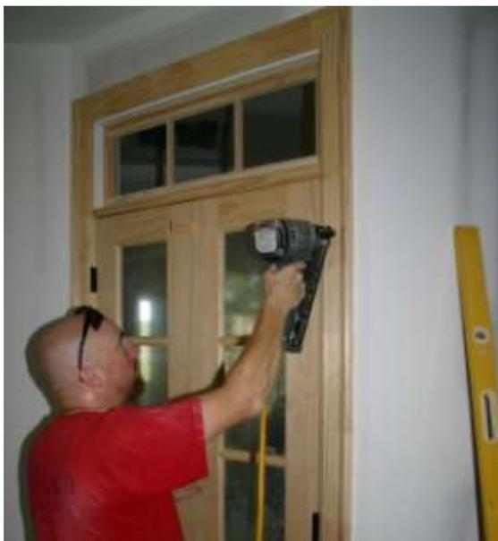
Once properly positioned, tack unit into place through casing
